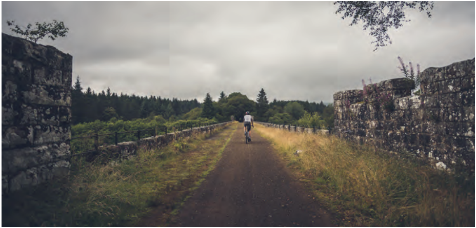
RIDING ON TOP OF KIELDER VIADUCT.
